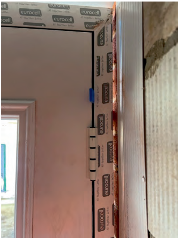
Gap on hinge side (max 4mm)
