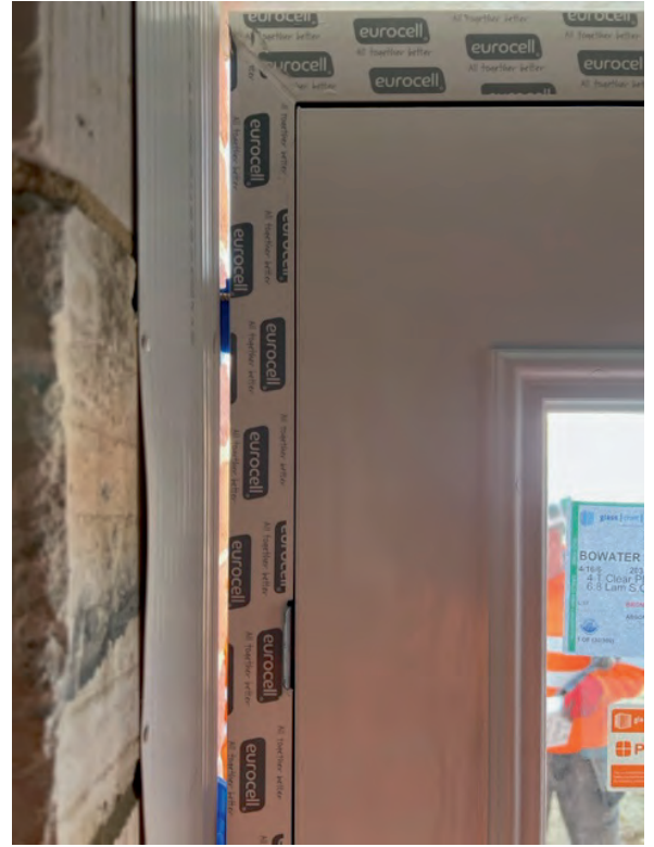
Gap lock side top of the door
