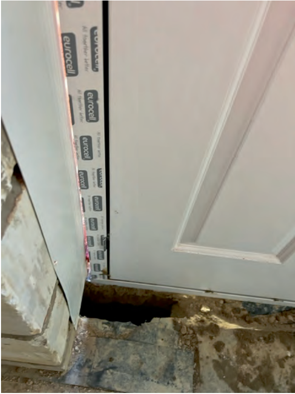
Gap lock side at the bottom of the door
