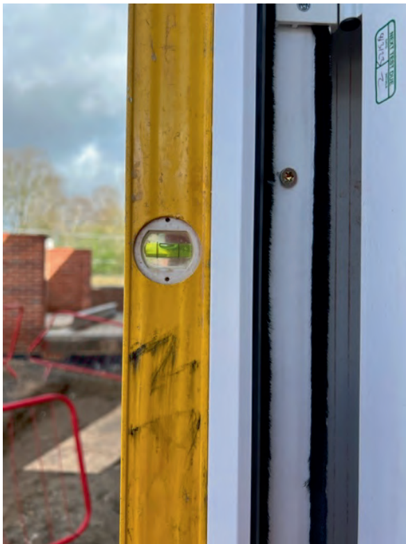
Hinge side level and plumb
